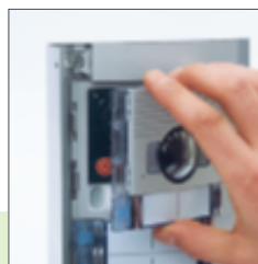
3 Loosen the clips and slip off the front plate
